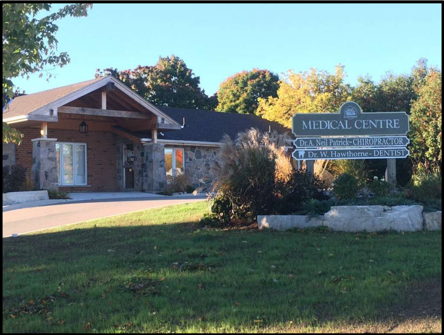
Renovated and expanded Creemore Medical Centre
